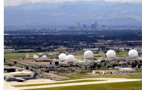
**Above:** The radomes on Buckley AFB, situated in clusters across the horizon, are large geodesic domes that contain satellite network tracking and intelligence equipment. Data collected is used to detect and report information on threats to the United States and allied nations. (U.S. Air Force photo)
