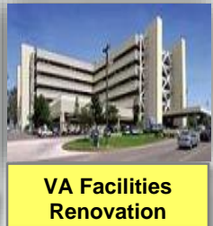
VA Facilities Renovation
