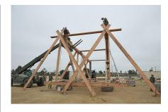
Above: Seabees assigned to Naval Mobile Construction Battalion 17 perform construction work on a 30-foot observation tower during a training exercise at Port Hueneme. (U.S. Navy photo)
