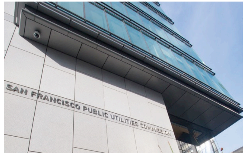
The San Francisco Public Utilities Commission building irrigates exterior vegetation using onsite water reuse.
