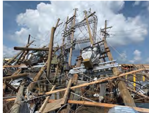
Energy infrastructure destroyed by Hurricane Ida in Louisiana
