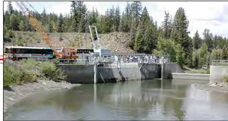
Azotea Tunnel Entrance
