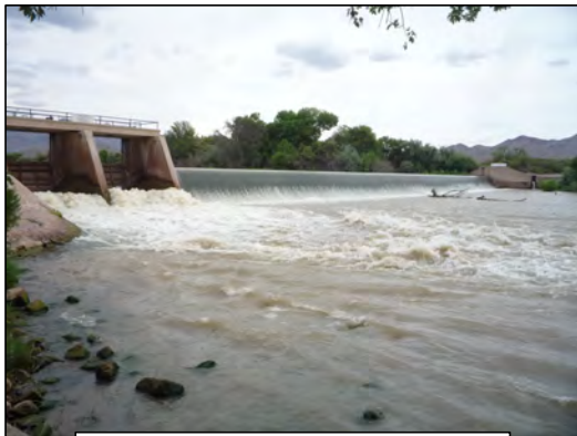
Percha Dam & Diversion
