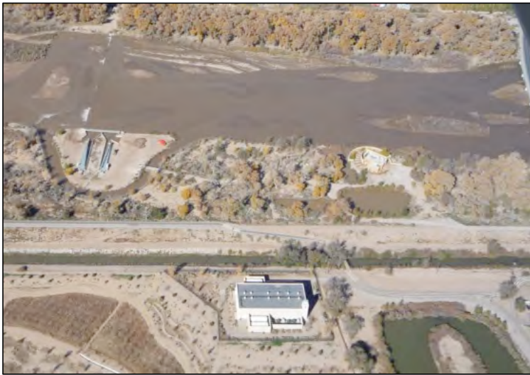
Diversion Dam & Pump Station
